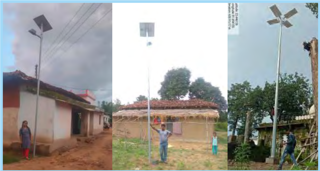
Solar Light Installation by MPCON under MPLDS/MLALADS Fund
